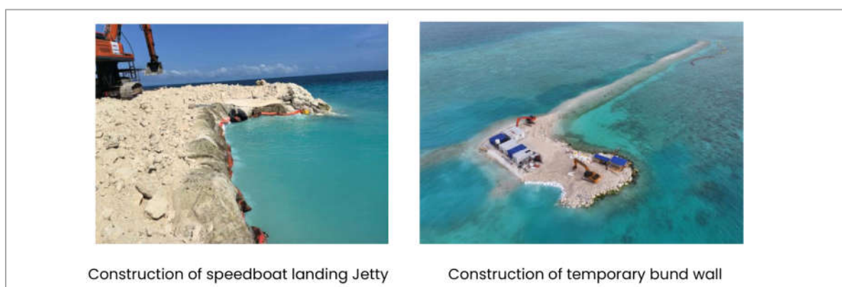
Figure 5: Extract from Contractor's progress report for the month of June 2025
